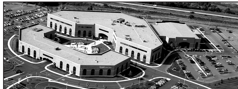
An aerial view of the 300,000+ s/f Integrated Health Campus.
